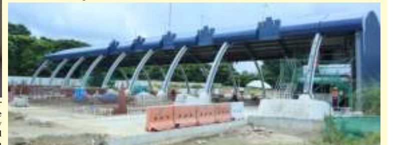
Governor's Drive Toll Plaza Construction progress
