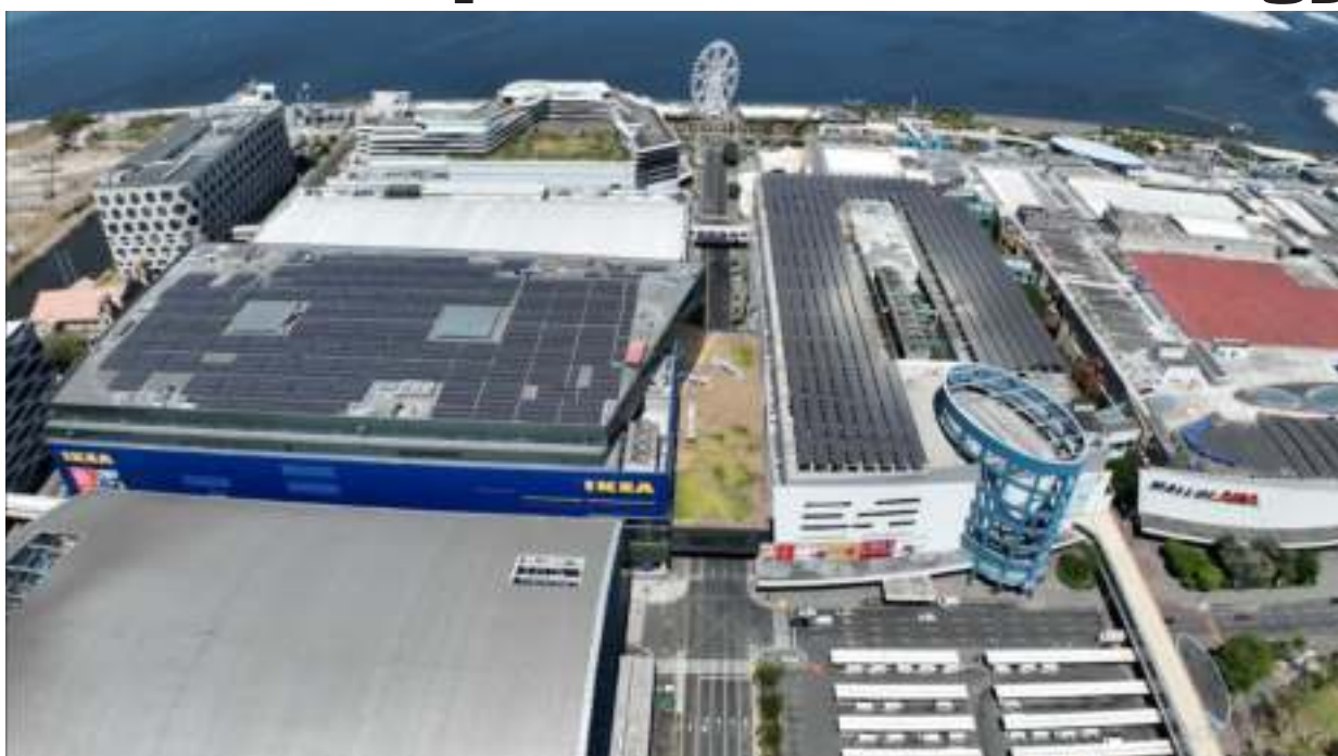
More than 3,600 solar panels were installed on the roof of MOA Square in the Mall of Asia Complex.
